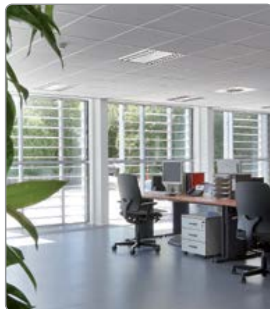
Loggia® 130 with Icarus® 125, TMWV Offices, Asse (BE)
