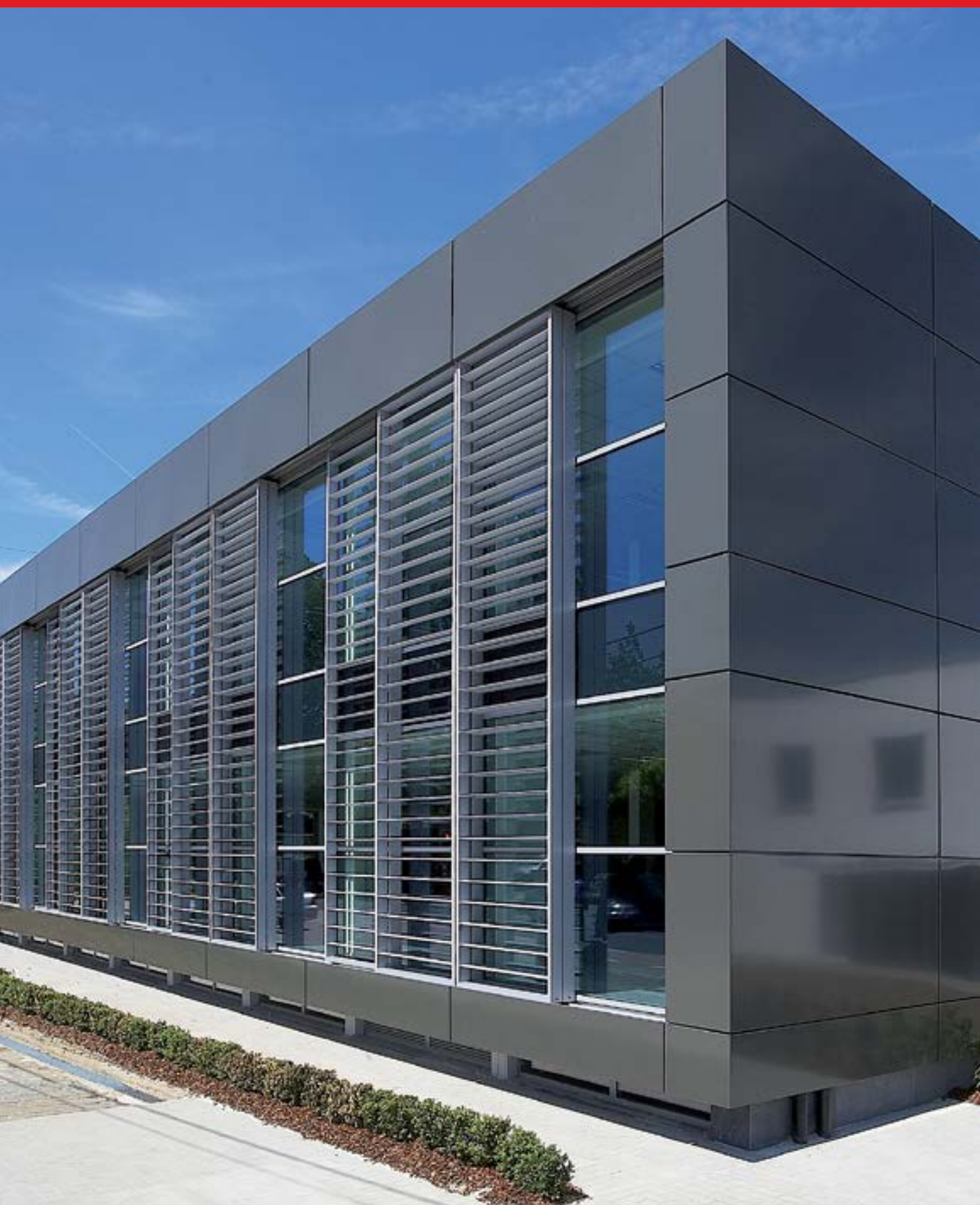
Loggia® 130 with Icarus® 125, TMWV Offices, Asse (BE)
