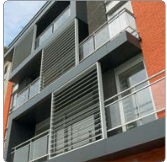
Loggia®, apartments, Kortrijk (BE)
